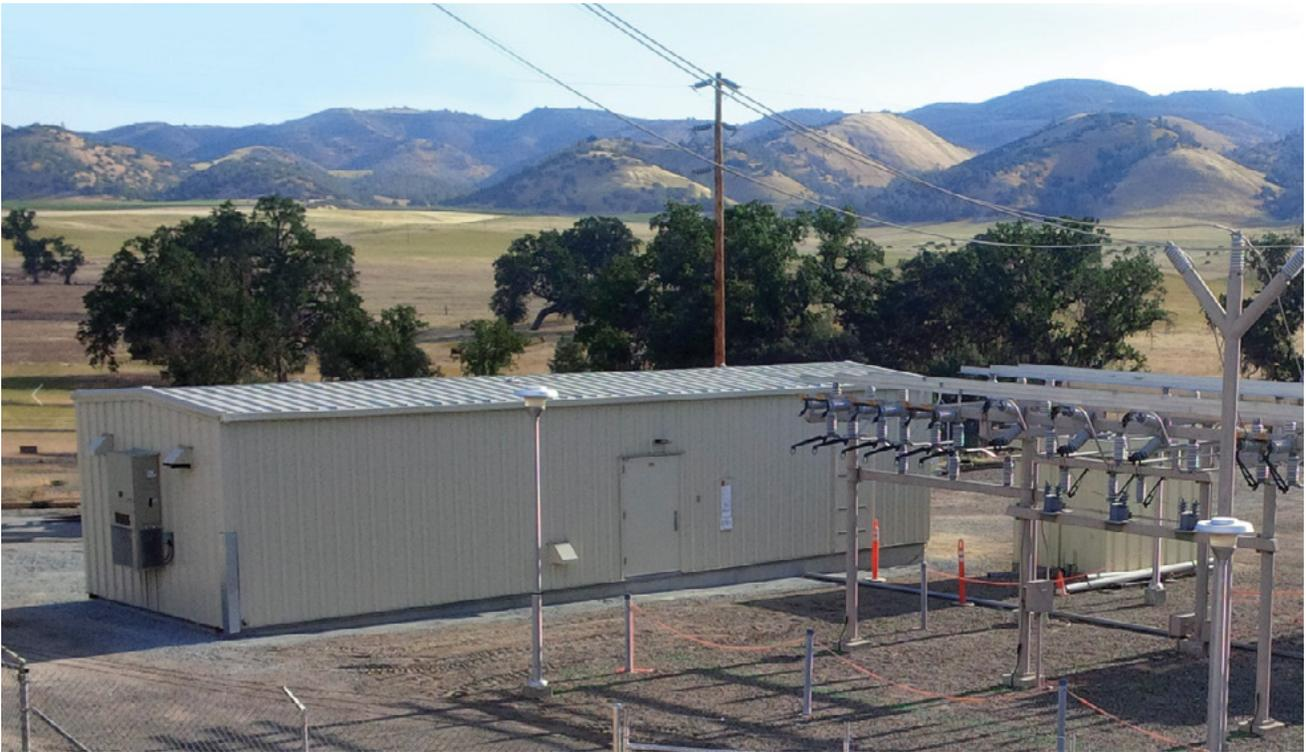
nVent TRACHTE buildings have house electrical and mechanical equipment preinstalled and tested before shipping for optimal project management, schedule efficiency & quality control.
