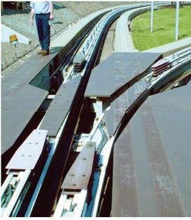
RAYCHEM Series Resistance heating cables provide the ideal solution for rail segments such as turntables and switches.
